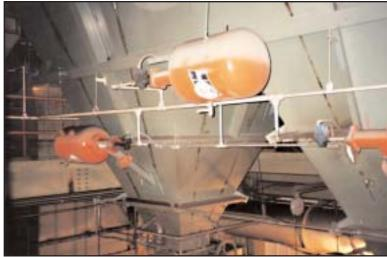
Figure 7. Unit 8 bunker pant leg air cannons
