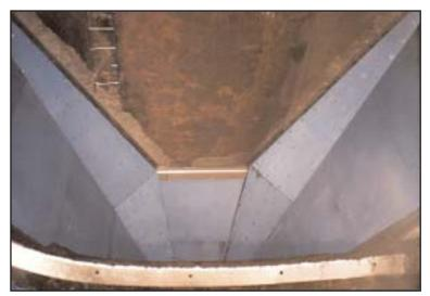
**Figure 10.** TIVAR<sup>®</sup> 88 liner installed on clean out plates and gunite sloping wall surfaces
